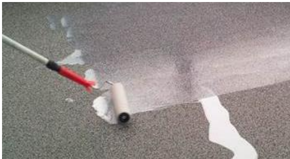
Image 3 and 4: application of the varnish
